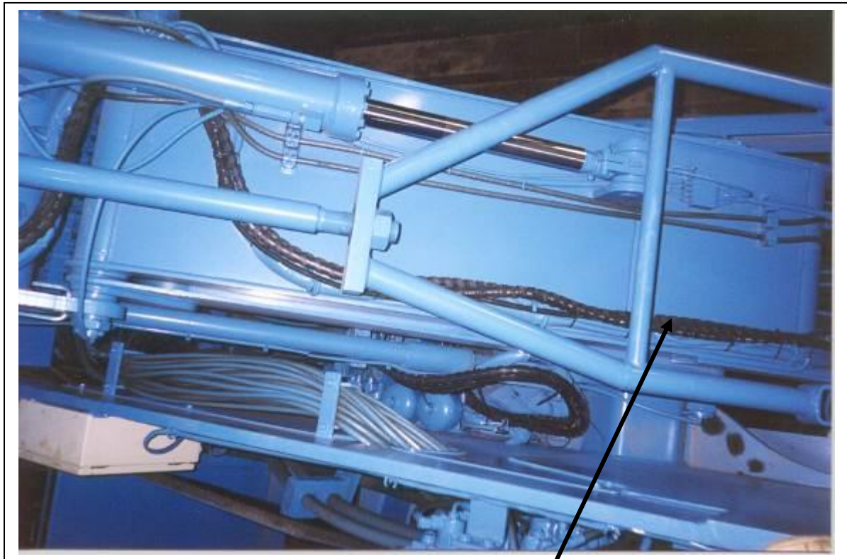
Hoses following factory wire bundle down to the cab.
